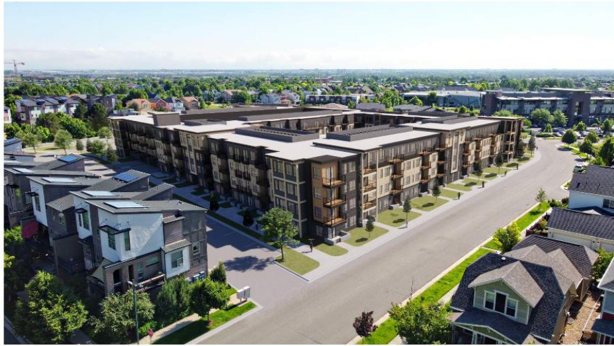
Aerial View From Southwest Corner
